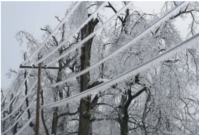
Figure 26 Ice Covered Power Lines
