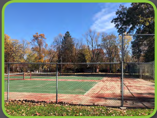
Tennis Courts in Need of Repair
