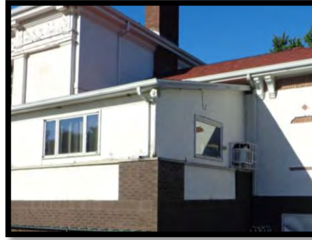
Pro Shop Window A/C
