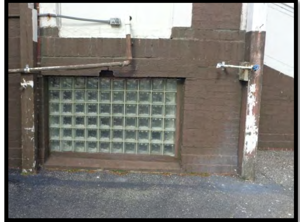
Outside Water Lines
