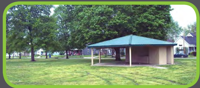
Shelter and Restrooms
