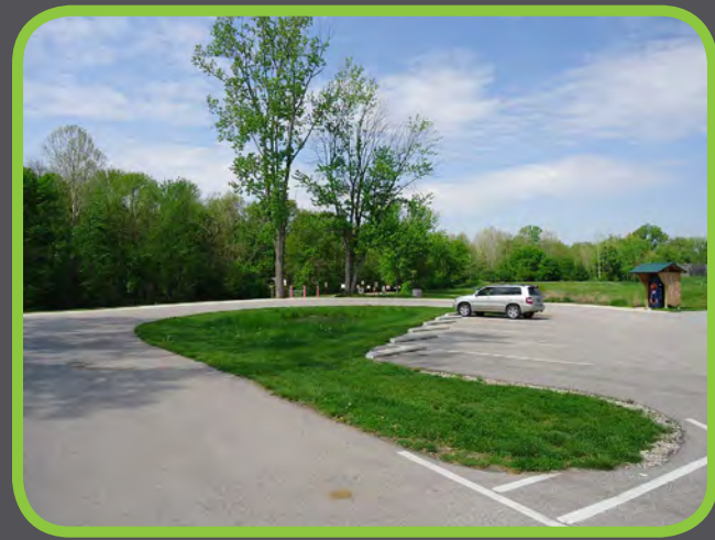
Jones Trailhead Parking Area and Bio-Retention
